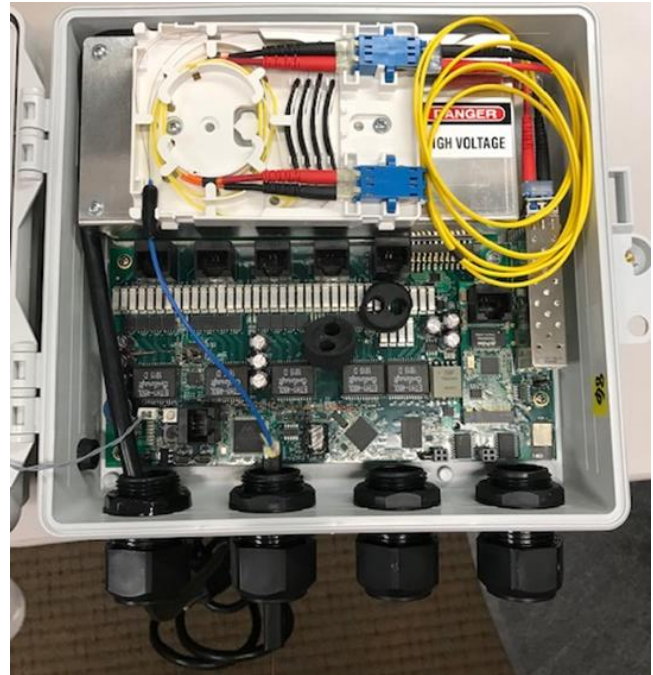
Fig. 6: Fiber Tray with Fiber Installed and Coiled
